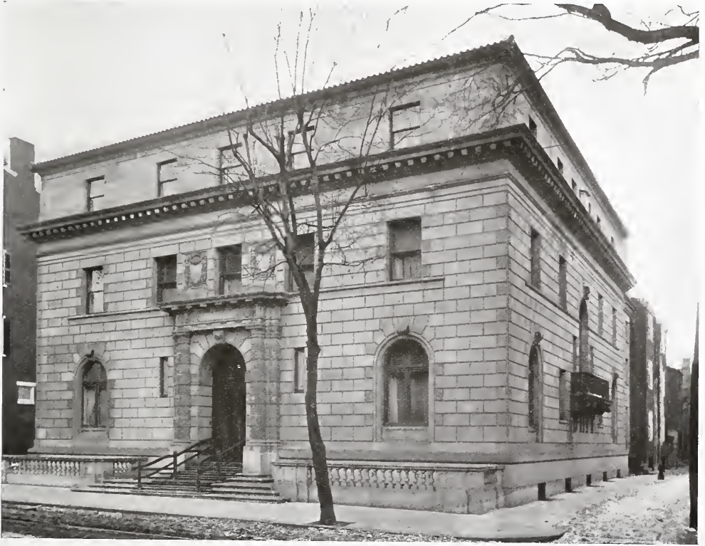
THE S. P. WETHERILL HOUSE.
